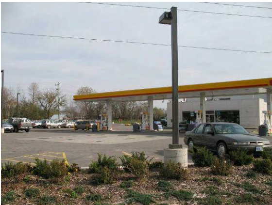
Photo 8 - 45: Southeast corner of Carlisle Road and Highway 6
